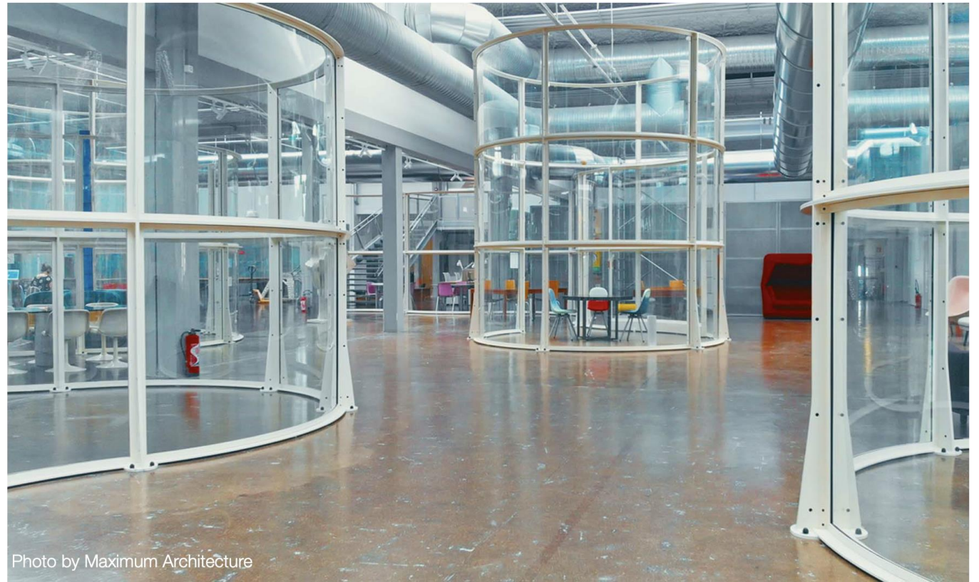
Internal partitioning walls in Papillon, Saint-Ouen by Maximum Architecture
