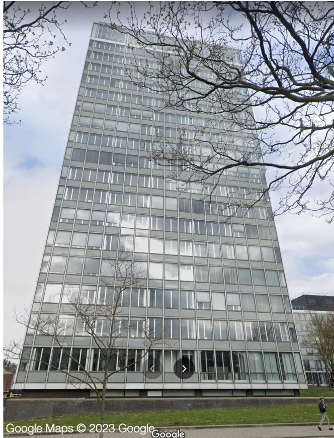
Curtain wall panels, The Hague
