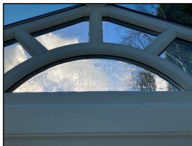
Fig. 3: Double glazed unit with single-silver coating showing internal condensation (Courtesy Pilkington | NSG)
