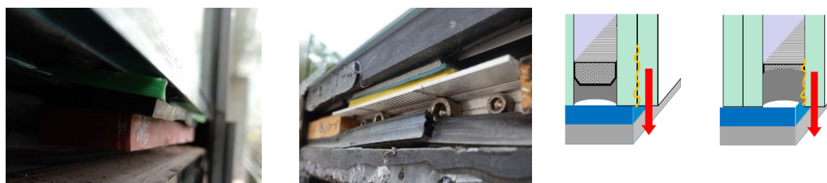
Fig. 6: Setting blocks, not properly installed.
