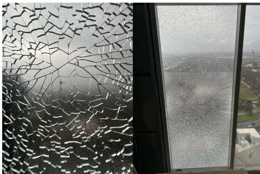
Fig. 3: Nickle Inclusion fracture on glass at jobsite.
