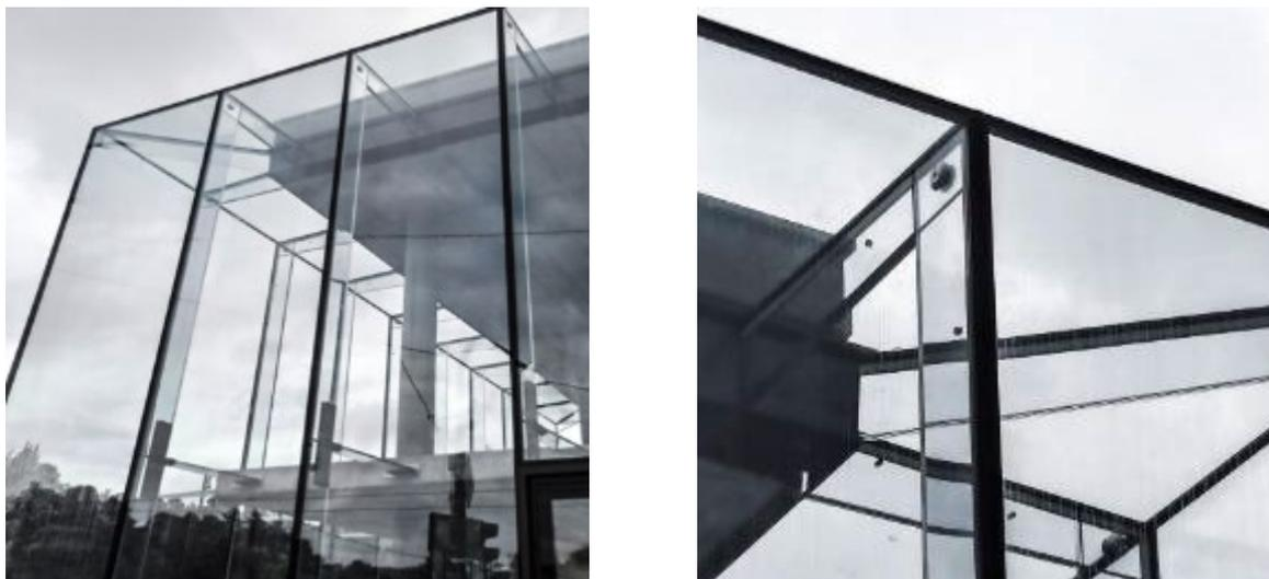
*Fig. 2: All glass construction with hybrid joints realised in Old Town Gate in Prague.*
