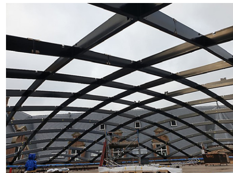
Figure 18: Left: installation of reciprocal frame ready, right: full steel grid installation ready.
