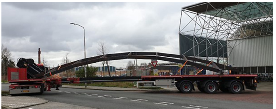
Figure 16: A green marked frame (see Figure 10) on transport.
