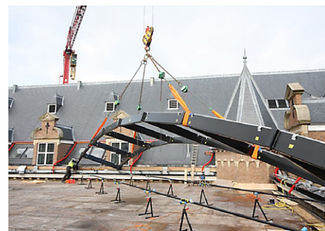
Figure 17: Left: hoisting a green frame, right: installing a green frame.
