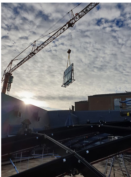
Figure 19: Left: hoisting of a stillage over the building to the loading platform, right: hoisting glass from the loading platform in its place.
