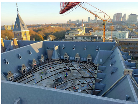
Figure 18: Left: installation of reciprocal frame ready, right: full steel grid installation ready.
