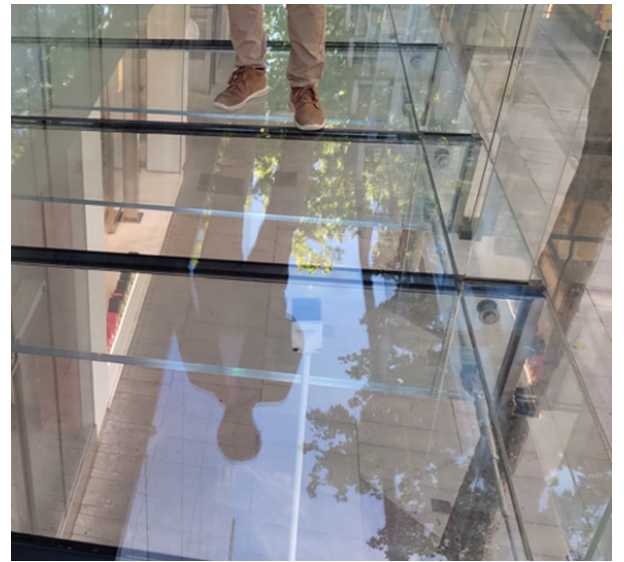
Figure 4. Final upper side of the canopy
