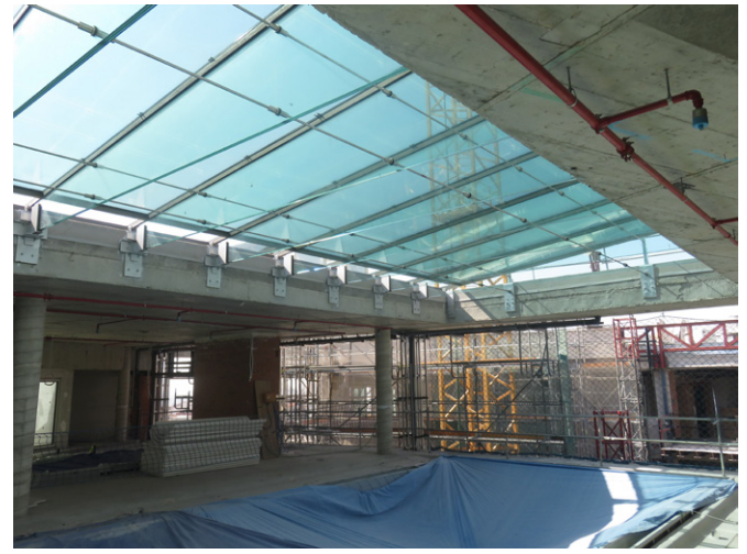
Figure 7. During construction. Skylight Hotel Four Seasons Canalejas.
