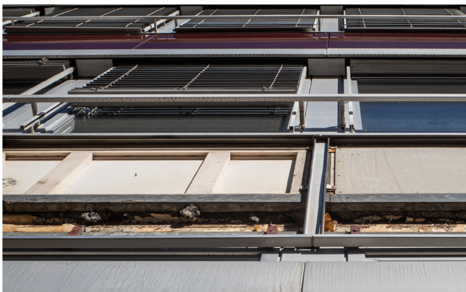
Fig. 5: Dismantling of glass cladding.
