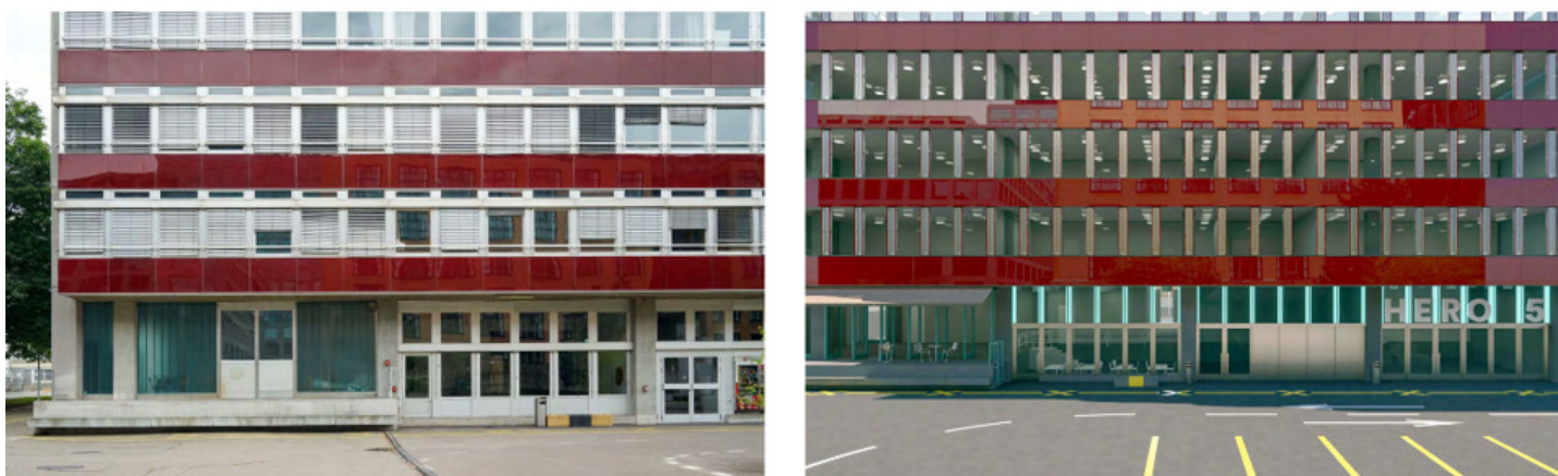
Fig. 8: Left: original façade, right: rendering of refurbished façade with glass reuse © Ekinçi Architekten GmbH.
