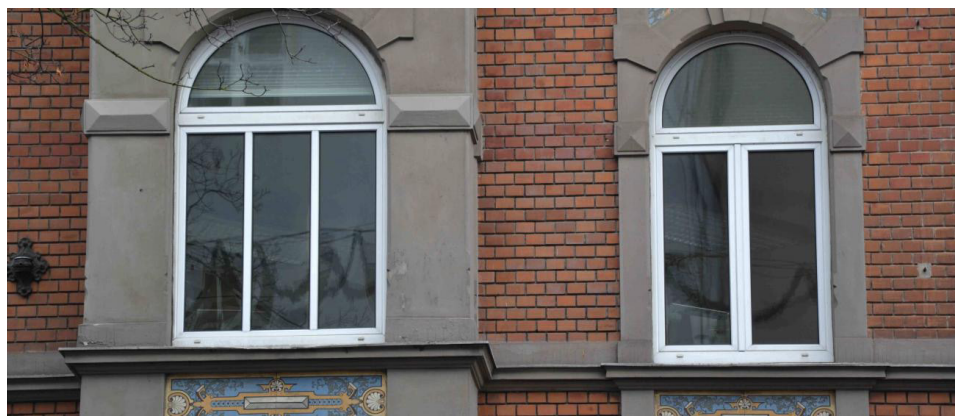
Figure 5 Plastic window frames in old buildings.
