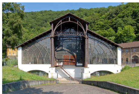
Figure 1 Sayner Hütte before renovation with historic windows (a) and afterwards with Floatglass (b).
