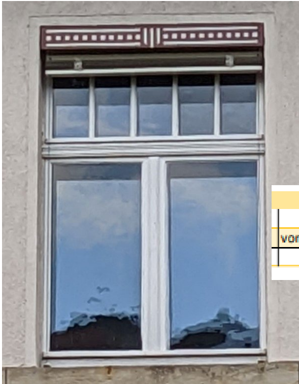
Window Wilder-Mann-Strasse 23c
