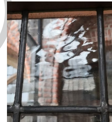
See-through drawn cylinder process. (Fourcault process). (Dralle).
