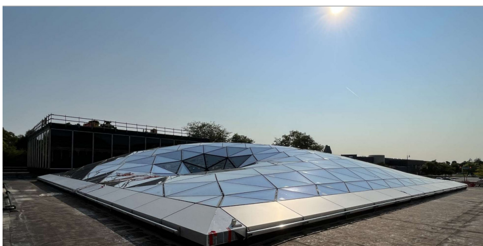
Figure 4: Roof structure from the outside (© Hahner Technik GmbH & Co. KG).
