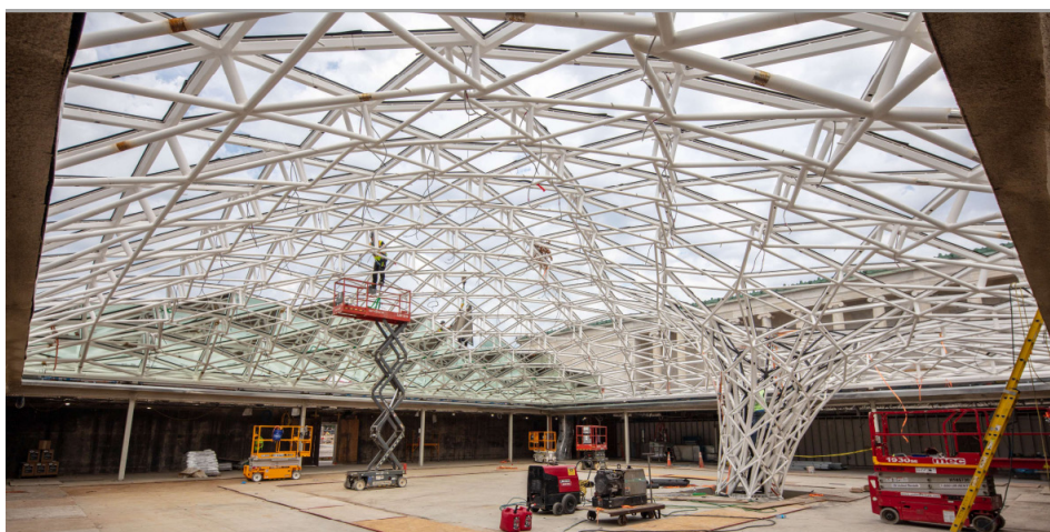
Figure 3: Roof structure during assembly from the inside (© Hahner Technik GmbH & Co. KG).
