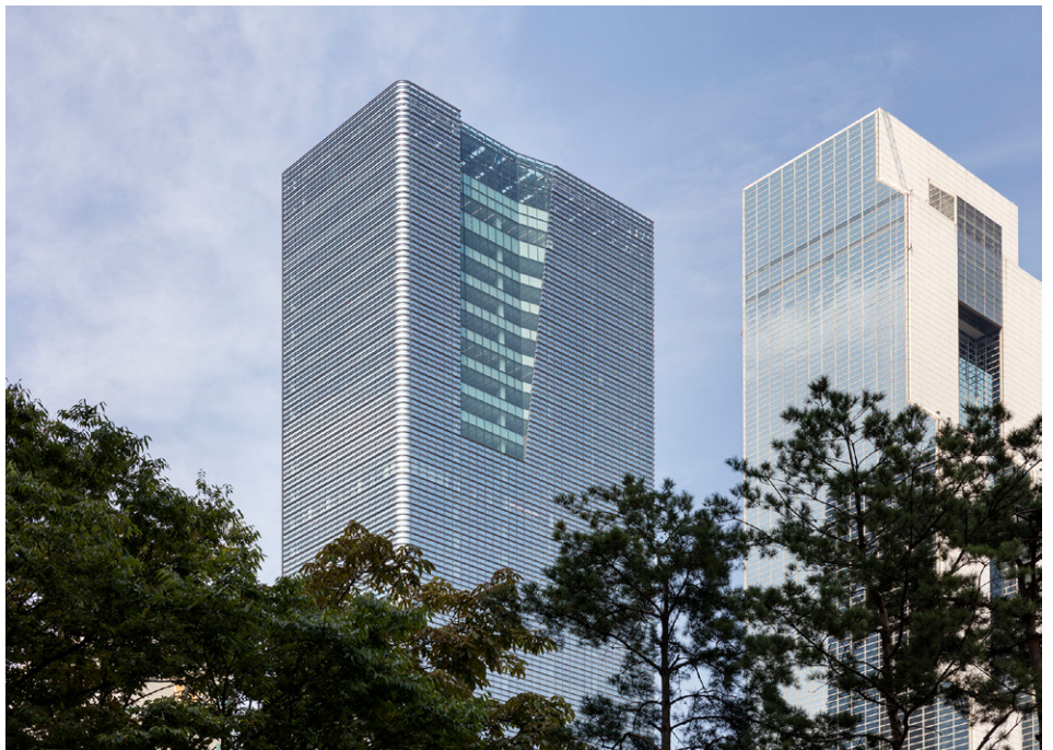
Figure 15: Parnas Tower (east elevation) with neighbouring WTC-Tower (© Namgoong Sun).
