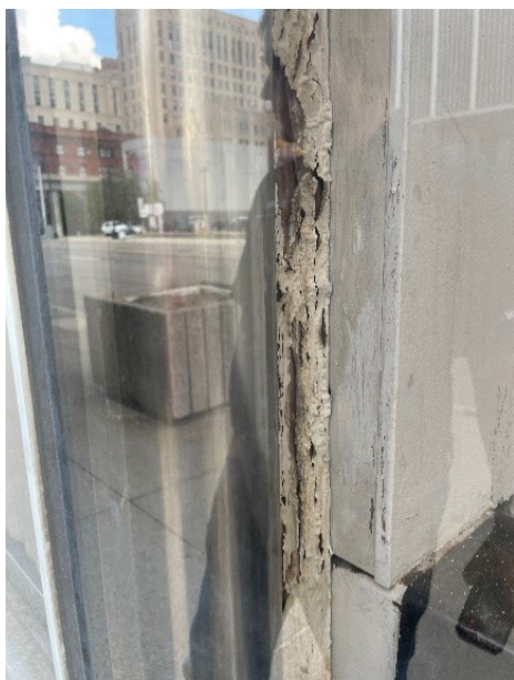
Figure 20. Degradation on interior acrylic coating that receives significant UV exposure. Courtesy of Dow.
