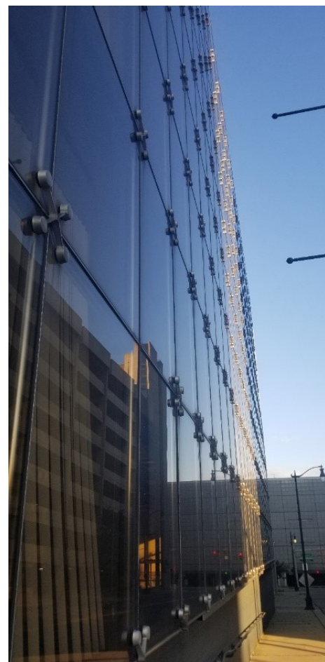
Figure 16. Missing Spider fitting shown on first row of glass lites – July 2021, Courtesy of SmithGroup.
