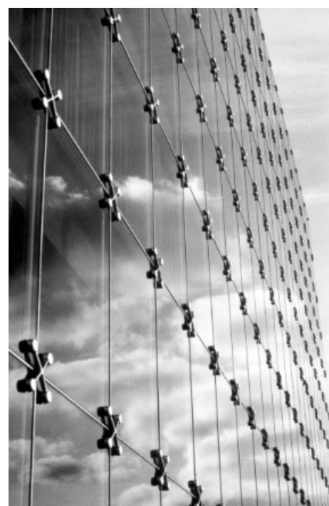
Figure 2. Typical Spider fittings. Photo courtesy of Dow.
