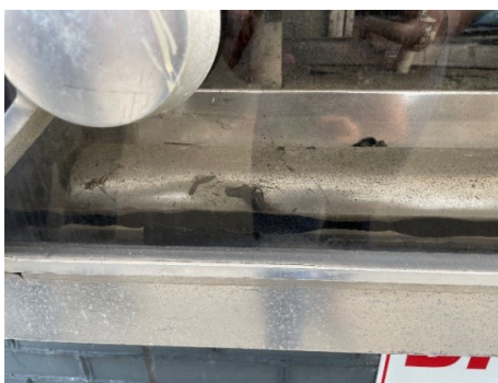
Figure 18. Smaller Bite dimension compared to original intent – July 2021. Courtesy of Dow.
