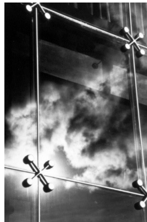
Figure 10. Cast aluminum Spiders deemed unnecessary in the system but added for additional safeguards. Photo courtesy of Dow.
