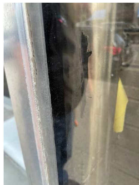
Figure 19. Appearance of smeared sealant – July 2021. Courtesy of Dow.
