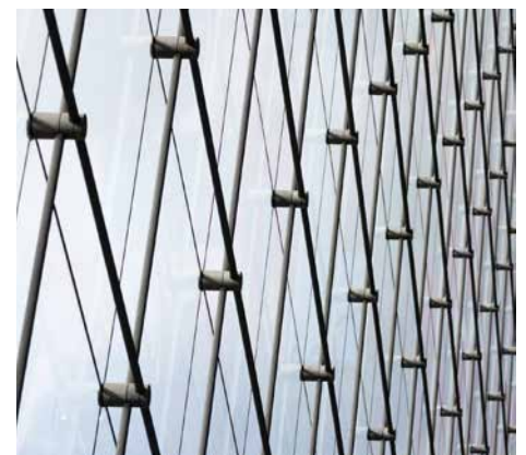
Fig. 19, 20: connections of the cable anchoring and the cable net
