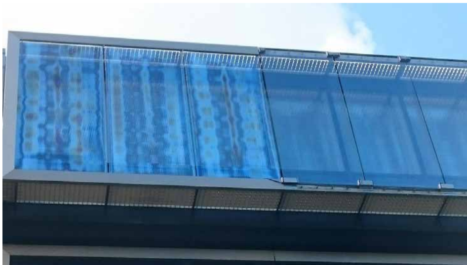
Figure 1 - Facade with tempered glass panes, left strong anisotropies and right low anisotropy, no polarising filters used (Luxembourg)
