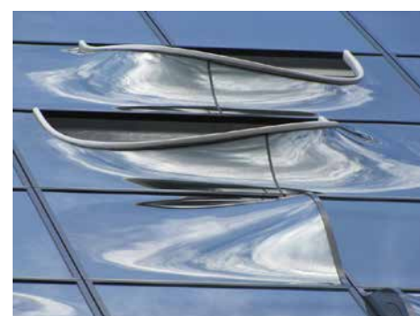
Figure 3 Double curved insulated glass units made of hot bent annealed glass, Concert Hall Elbphilharmonie, Hamburg (Germany)
