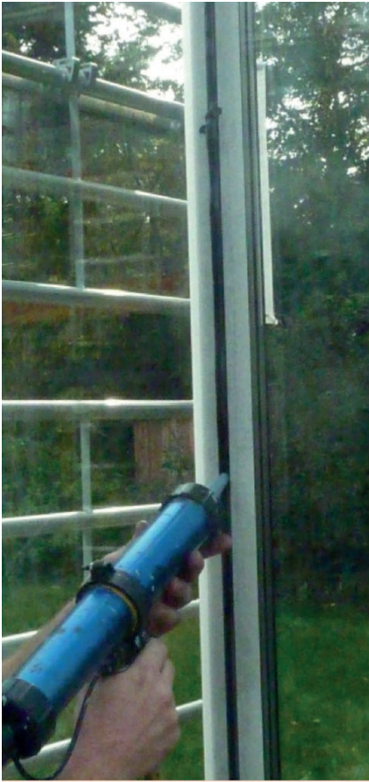
Fig. 7a) and b) Sealing of glass wall joint and finished façade (www.master-ateliers.com)
