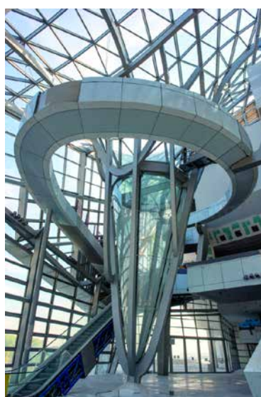
Figure 2 (right) Free-formed hot bent annealed glass, Musée des Confluences, Lyon (France) ©Karin Jobst
