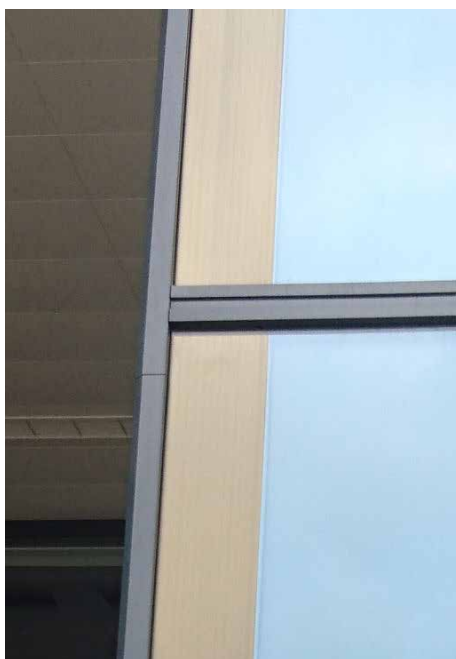
Fig. 1: Edge-printed coated glass with typical colour drifting
