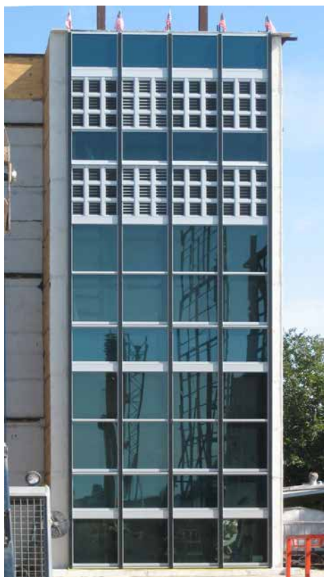
Figure 11 Spandrel glass reflection exceeds that of vision glass.
