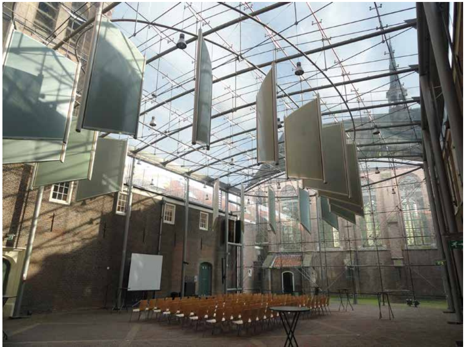
Fig.6: Prinsenhof museum hall, Delft, with glued Quattro connections in roof and facades.
