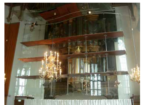
Fig. 30: Curved glass curtain in front of the 17 th century organ which will be made sliding sideward.
