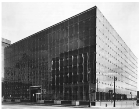
Figure 1: 455 W Fort Street, Detroit, the world's first four sided silicone structural glazing project, 1971 designed by architects Smith, Hincham and Grylls. Photo courtesy of SmithGroupJJR
