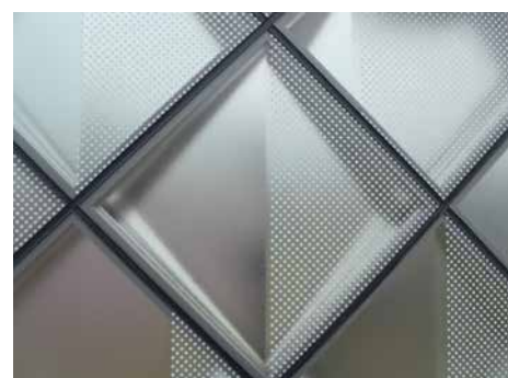
Figure 5 Close-up of 1:1 mock-up with dry gaskets instead of wet sealed joints © Richter Musikowski Architekten
