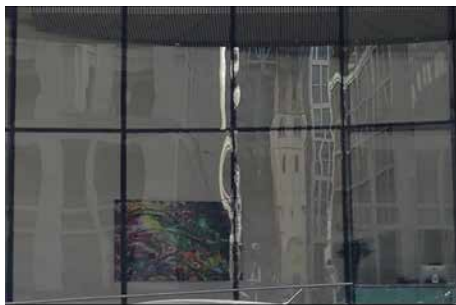
Figure 2: Distortion between curved panels
