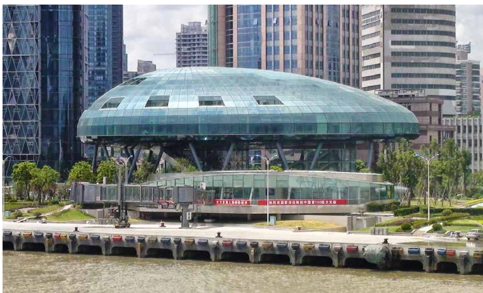
Figure 6 Shanghai Ocean Terminal, planar-quad glass panels because of its homothetic surface
