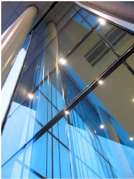
Fig. 16: The experimental façade with the vertical Aramid cables inside of the IGU inner space.
