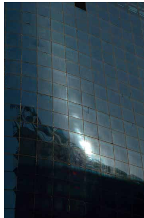
Figure 03: Free-form shape cold-bent structural silicone glazed façades (partially hot bent-glass is used)
