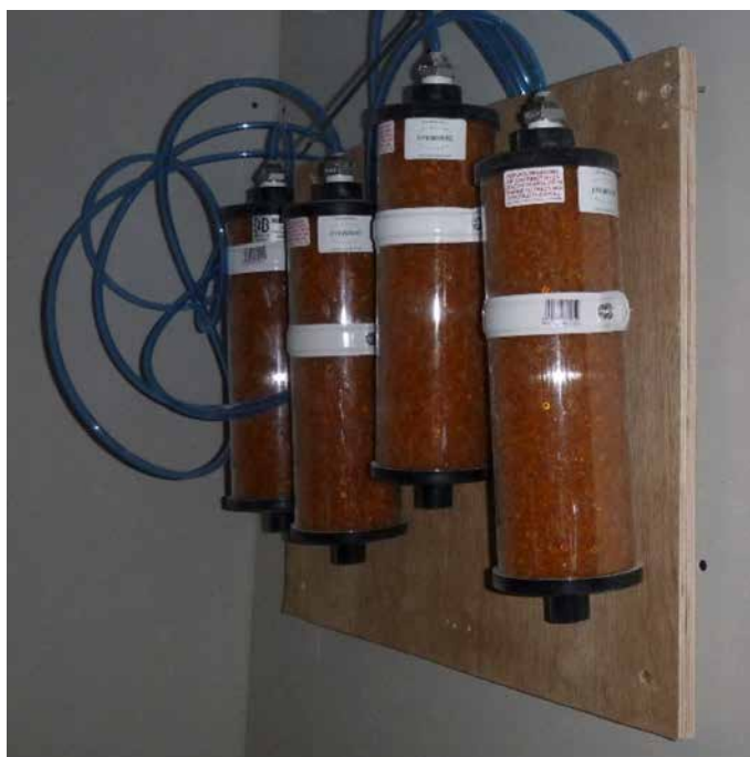
Fig 4 Desiccant breathers installed
