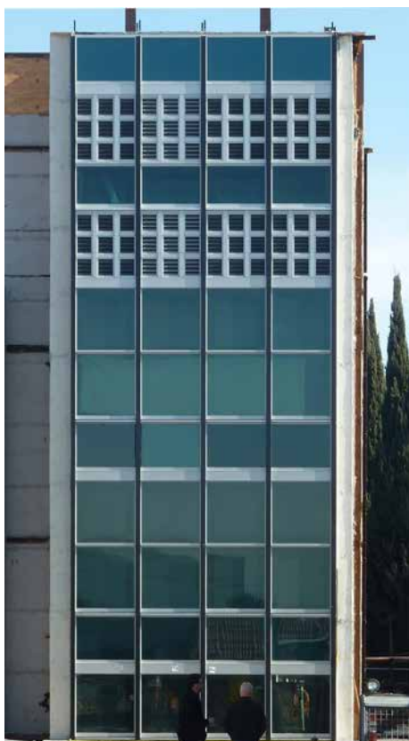
Figure 12 Trials of spandrel glass options with reduced reflectivity. From left to right along middle spandrel glass options: (1) simulation of historic monolithic glass, (2) insulating glass with clear inner lite, (3) and (4) insulating glass with gray inner lite and low-e coating. Note that appearance of (1) matches (3) and (4).
