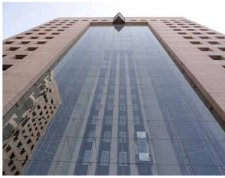
Fig. 4,5: Inside and outside of the OZ building with 52 x 16 m Quattro glass façade in Israel.
