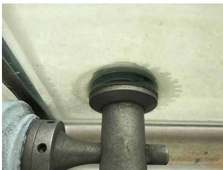
Figure 7 Delamination around point support fitting
