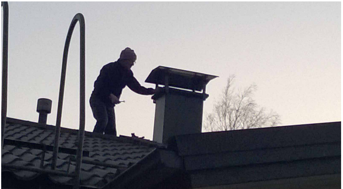
Figure 2. Assembling the chimney cover [Photo: Olavi Uusitalo].
