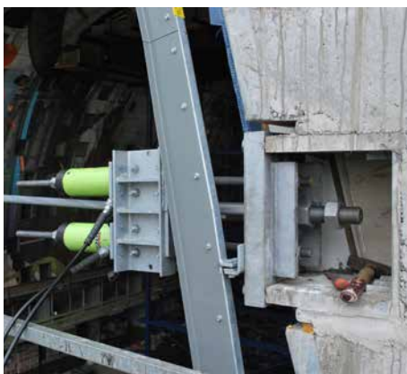
Fig. 19, 20: connections of the cable anchoring and the cable net
