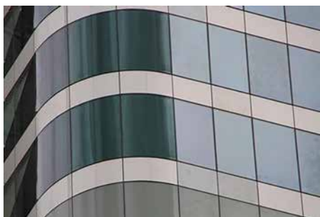
Figure 3: Inconsistency in coating colour
