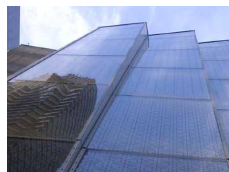
Figure 4 Cold bent insulated glass units (4th point out of plane), Singapore Chancery, New York (USA)
