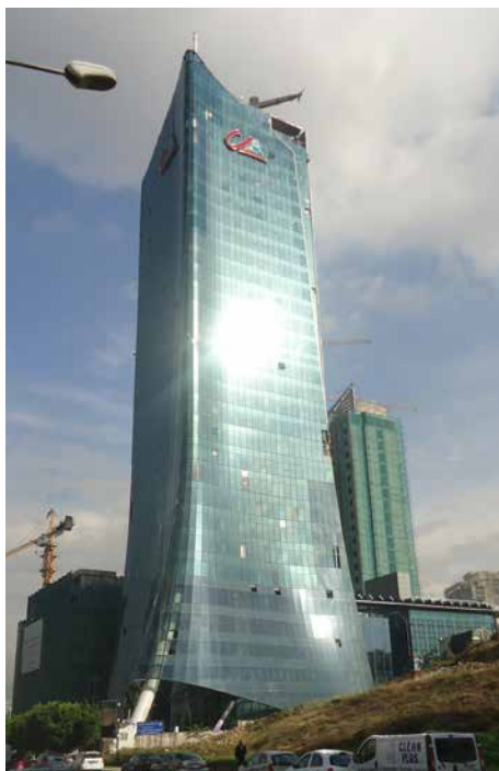
Figure 02: Single corner cold-bending structural silicone glazed façades, Credit Libanais, Beirut
