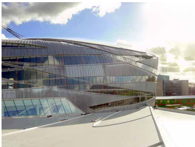
Fig. 10,11: Back side of the town hall with the cold twisted insulated laminated glass panels
