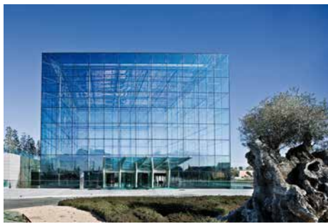
Fig. 8, 9: outside and inside of the glass cube with slender cable structure stabilisations
