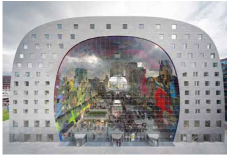
Fig. 17, 18: the Market hall with 2 x 700 mm deformation due to maximum wind loading.
