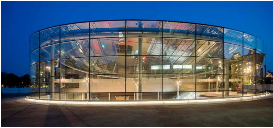
Fig. 25: The cold bent glass facades of the Van Gogh Museum entrance forms a regularly curved facade
