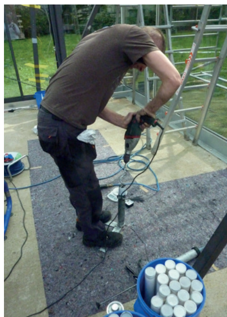
Fig. 6a), b) and c) Blending, controlling and documentation for each cartridge during on-site-bonding
