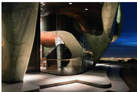
Figure 5 Double curved hot bent annealed glass, Baha'i Temple of South America, Santiago de Chile (Chile) © Jose Luis Stephens
