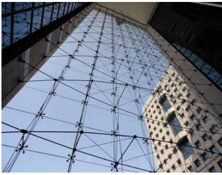
Fig. 4,5: Inside and outside of the OZ building with 52 x 16 m Quattro glass façade in Israel.
