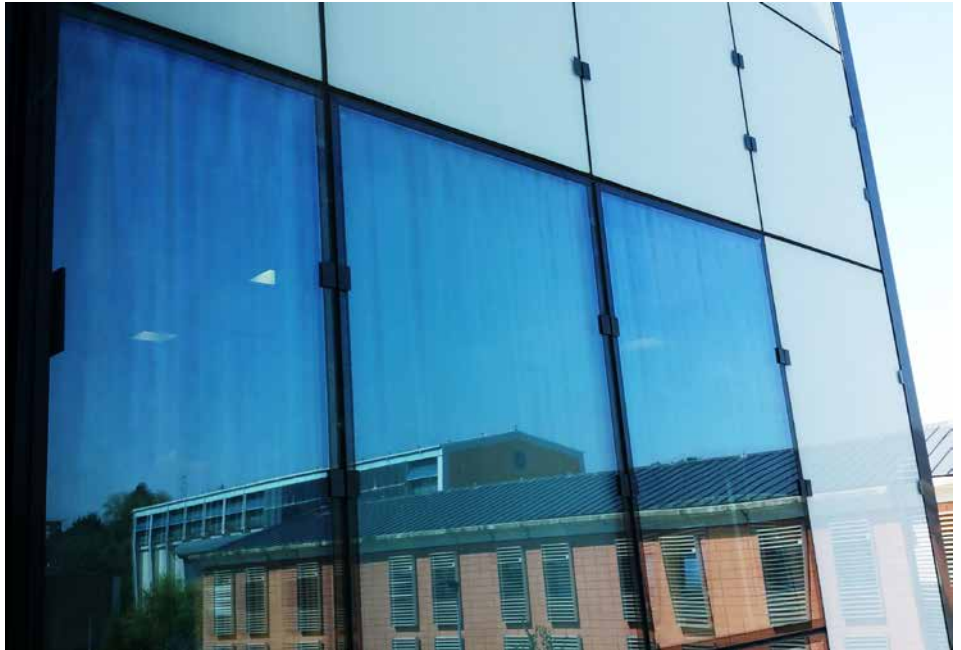
Figure 1 Anisotropy visible on a façade.
